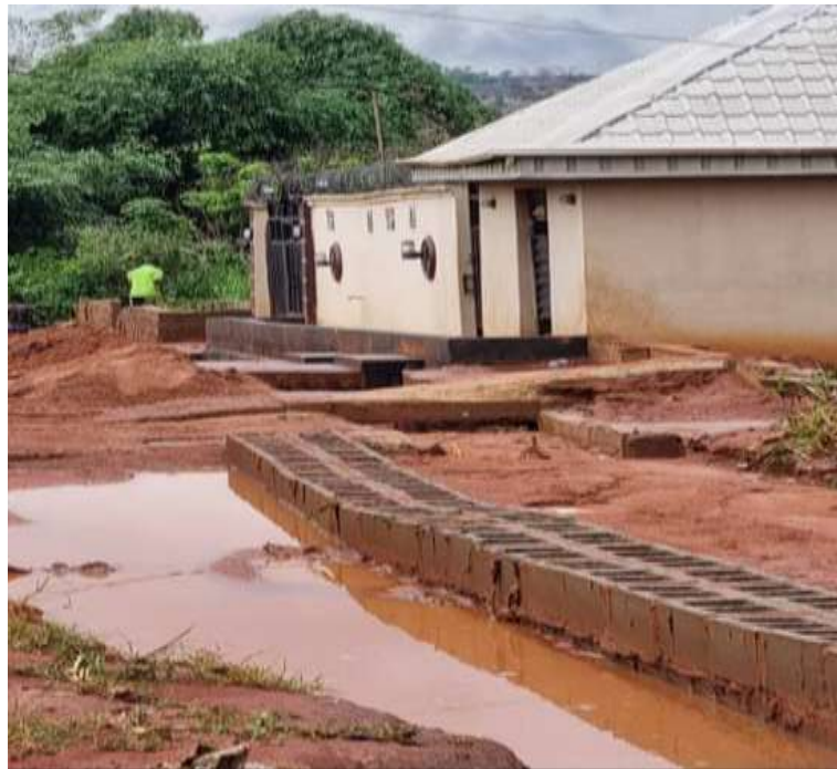
Figure 3: A residential house built on a flood plain without a proper drainage system at Ogun State
