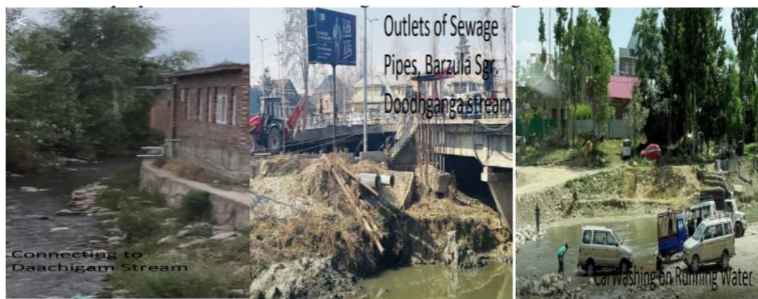
Figure 4. Improper House Hold Waste Management and Drainage Issues
