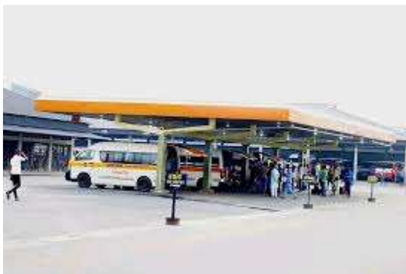
Figure 1. AKTC Park Terminal, Uyo
