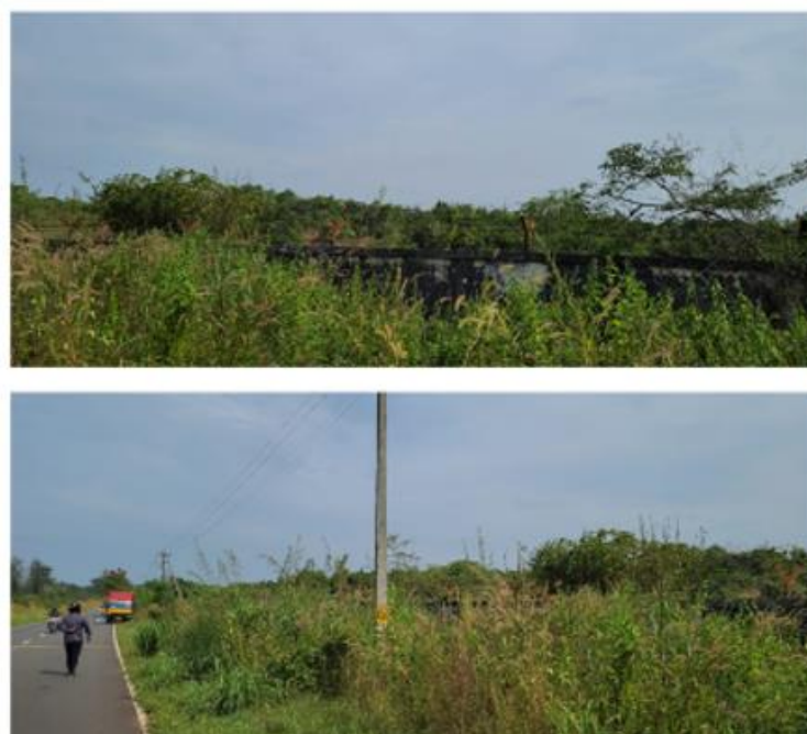
Fig. 6 Existing Condition of Cheemeni IT Park SEZ
