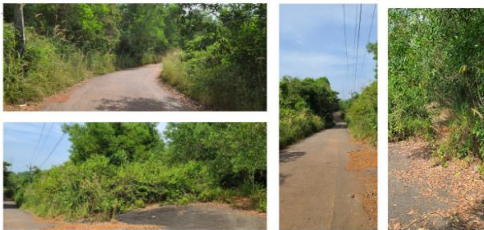
Fig. 5 Existing Condition of Eramam IT Park SEZ
